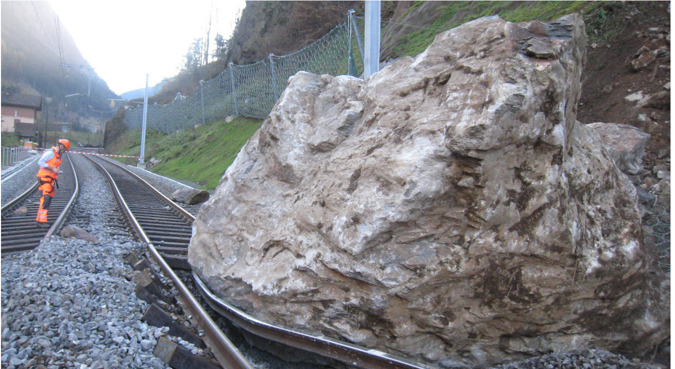
Abb. 4.2: Felssturz vom 14. November 2012 (Foto: SBB AG) Rockfall event on 14 November 2012 (Swiss Federal Railways)
