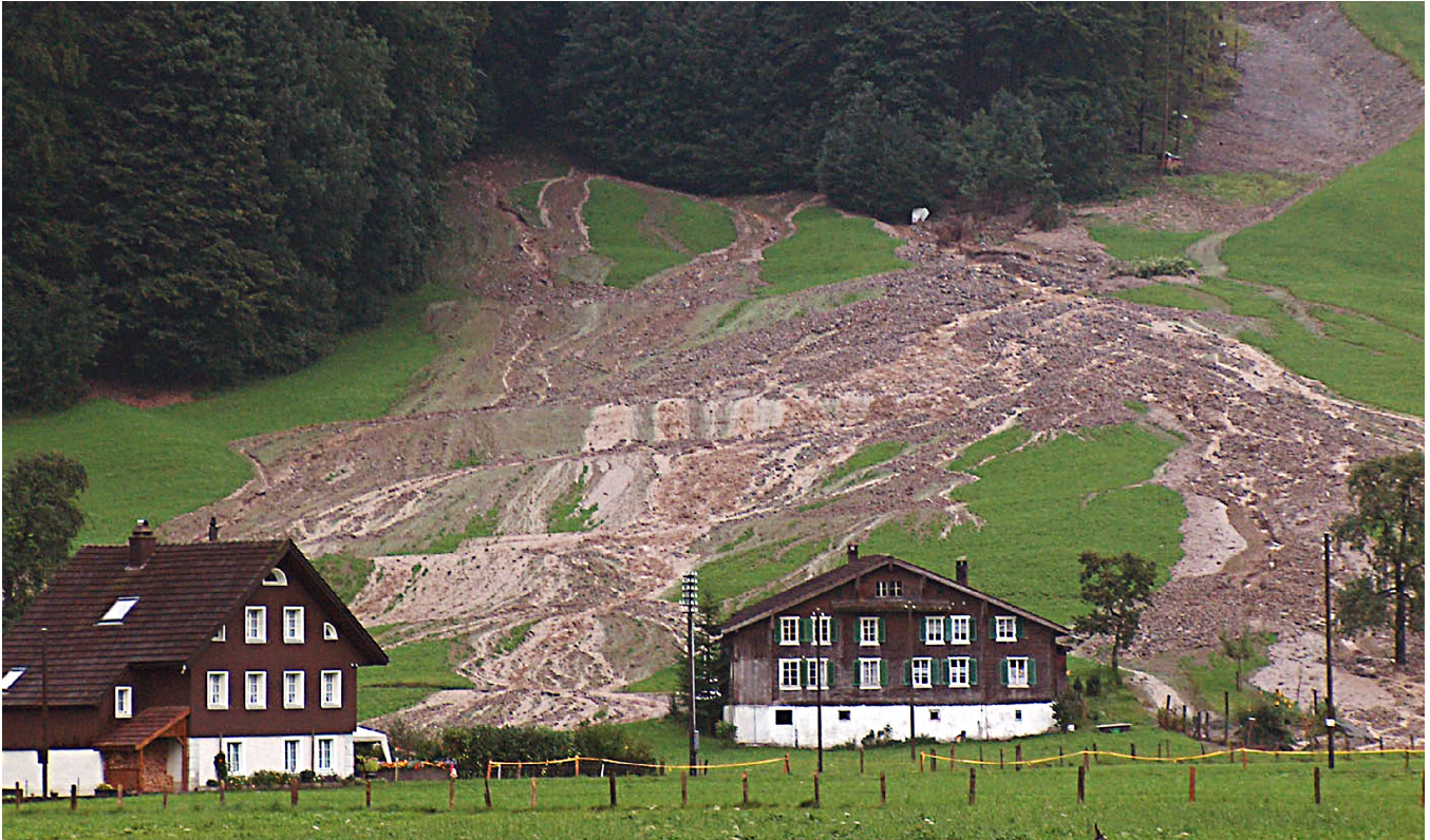
Schadarme Überlast des Humligensammlers. Overflow of the retention structure in Humligenbach did not incur significant damage in the overflow area
